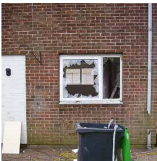
Empty home prior to intervention
